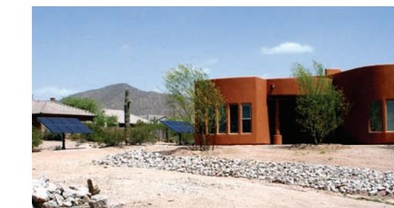
This residence is a new, custom-built ZERO-Energy home with many energy saving features – including a 3.2 KW PV array with dual-axis tracking and a solar water heating system.
