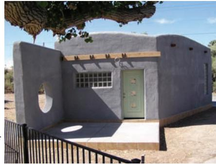
This 500 square foot office structure is constructed of 4 tons of waste paper mixed with other materials to provide a low-cost high insulation prototype building material. The facility, which cost about half what conventional construction costs, is expected to consume about 70 percent less electricity and includes monitoring devices for power usage and various structural elements of the building.
