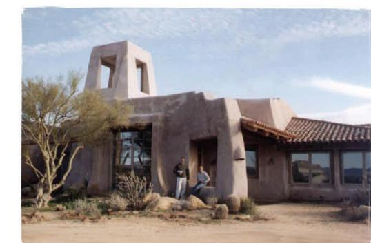
This super-insulated (R50 walls, R67 attic) builder's strawbale home has it ALL. It incorporates a plethora of passive and active energy-saving strategies—including orientation, energy efficient windows, structure shading wing walls, thermal mass plenum floors, cross ventilation, a cool tower (gravity driven evaporative cooling system) and more. A grid-tied PV system supplies electricity for the super-efficient appliances and greywater reclamation waters the veggie garden.
